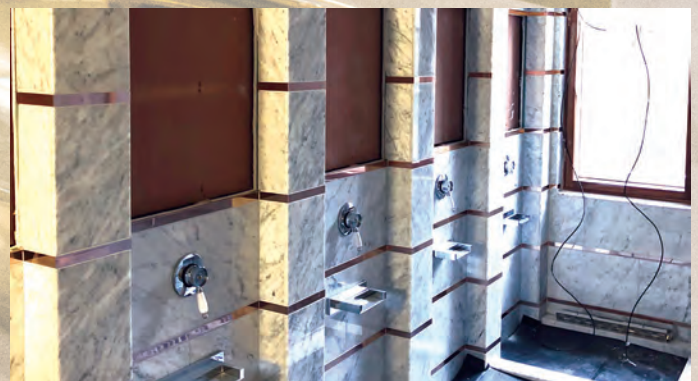
Installation of wudu stations
