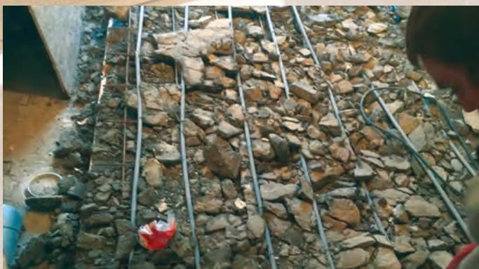
Installation of underfloor heating
