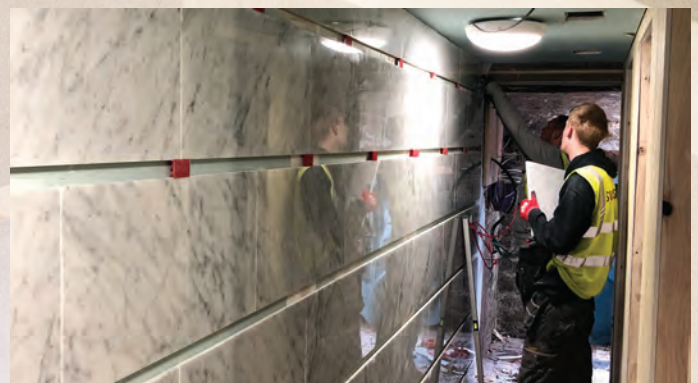
Installation of marble stone wall tiles
