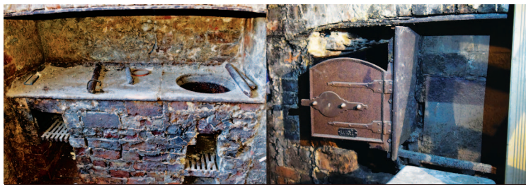
Restoring original Victorian kitchen into Cafeteria. Image shows original Victorian bread making stove and cooker.
