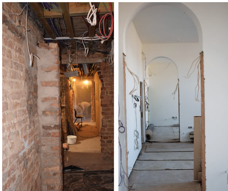
Training rooms all to be completed with lime plaster incorporating horse hair as with listed building requirements.
